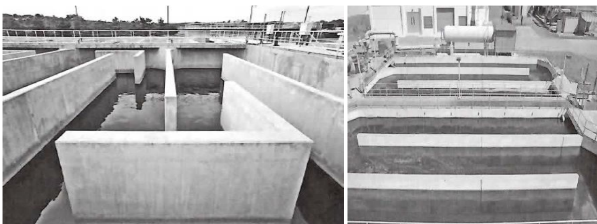
Figure 35 Examples for chlorine contacts basins: left serpentine plug-flow basin, right with rounded corners; adapted from Asano et al. (2007) – Design can be adapted for PFA contact basins
